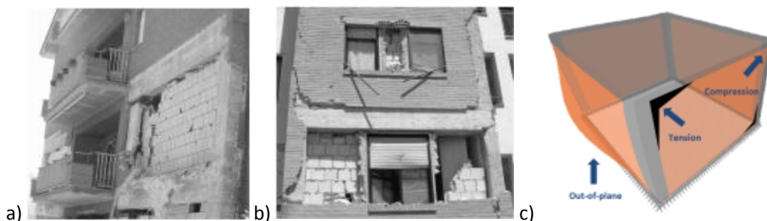
Figure 1: In-Plane (a) and Out-of-Plane (b) failures and their schematic visualisation (c).
